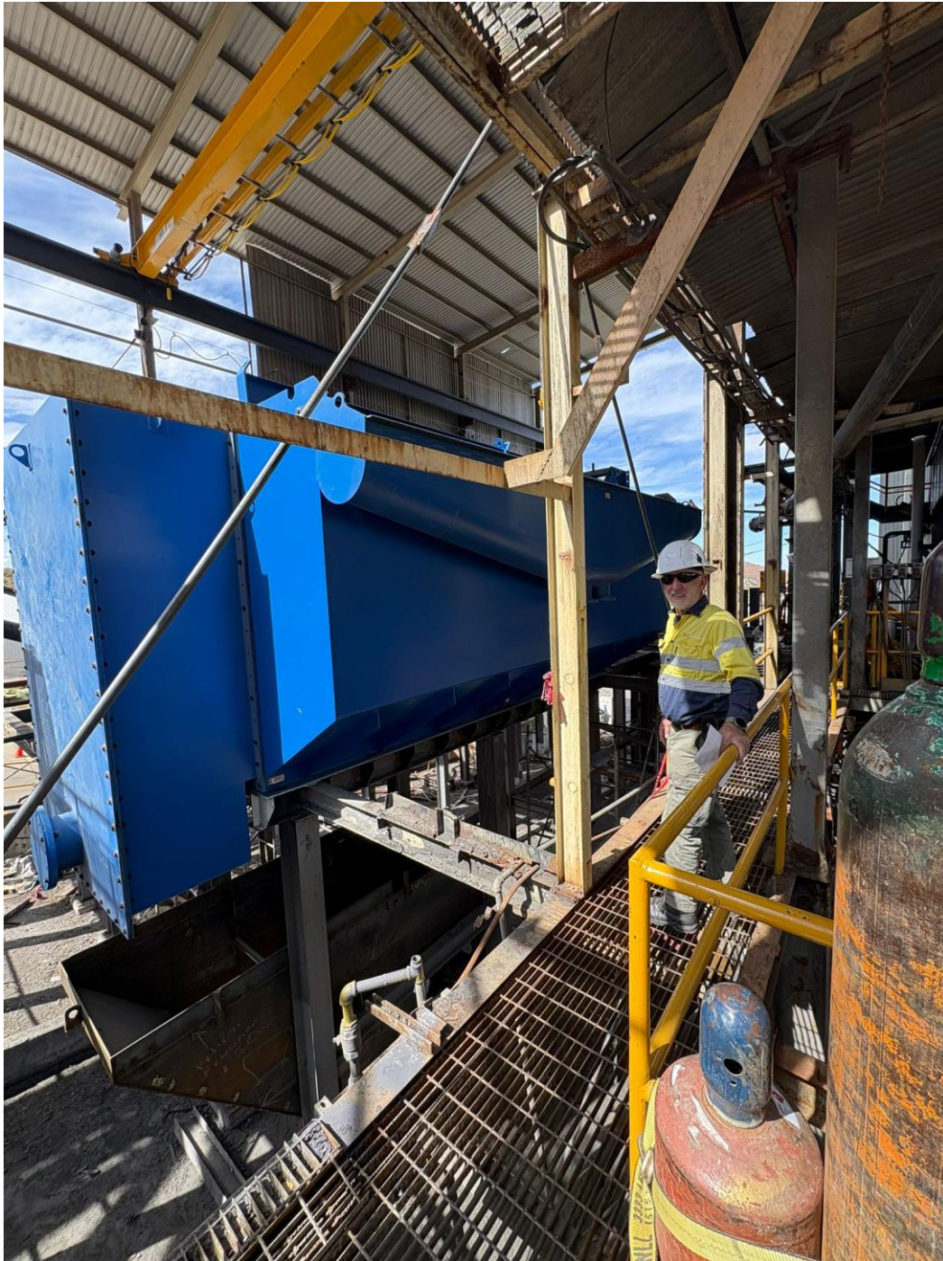
Figure 2: Installation of the new flotation cells is underway
